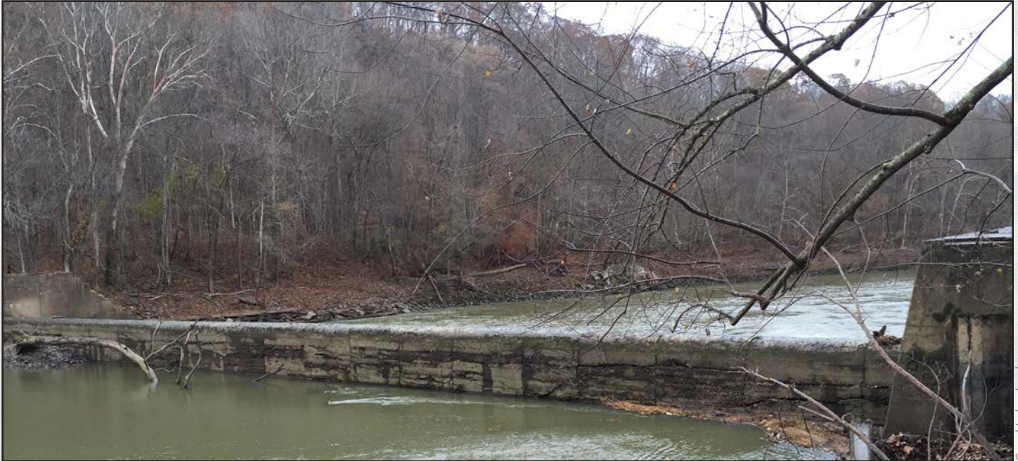
Pictured above is a segment of the upstream face of ogee weir dam.
