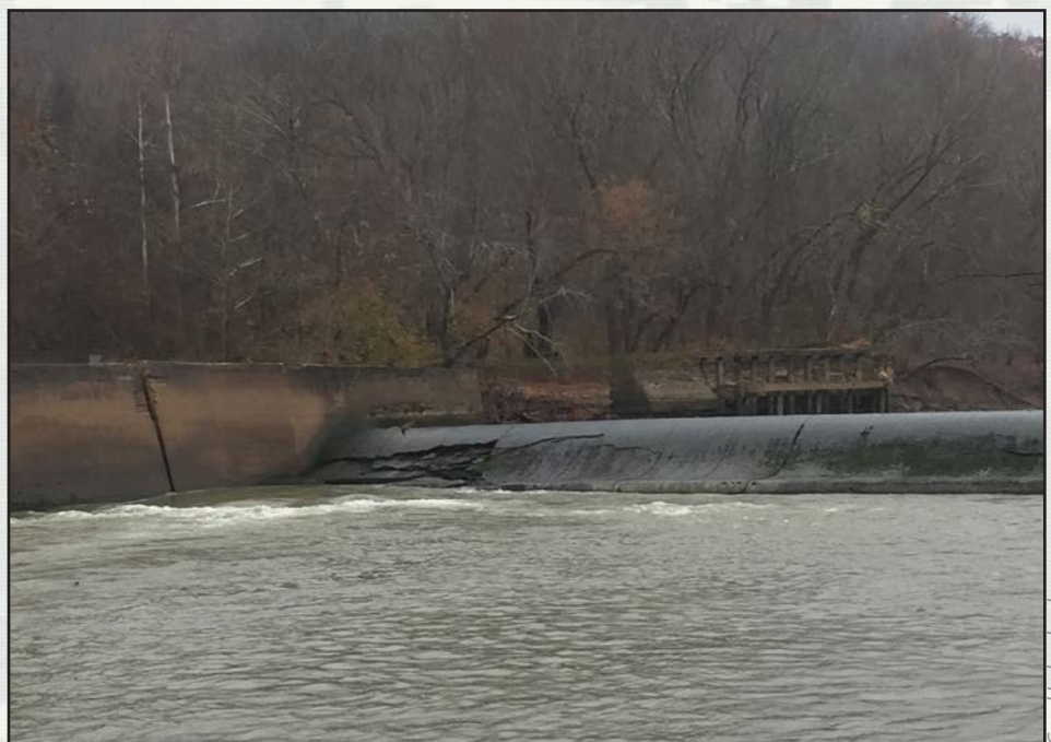
Pictured here is the downstream face of the Ogee Weir Dam. Note under flow of Green River at interface with the Lock Wall.
