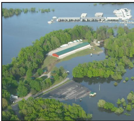
An aerial shot of Nolin River Lake in Bee Spring, Ky., shows record water levels around the Moutardier Marina and boat ramp access areas. Nolin Lake was one of five Louisville District lakes that reached spillway level during the flooding event in May.
