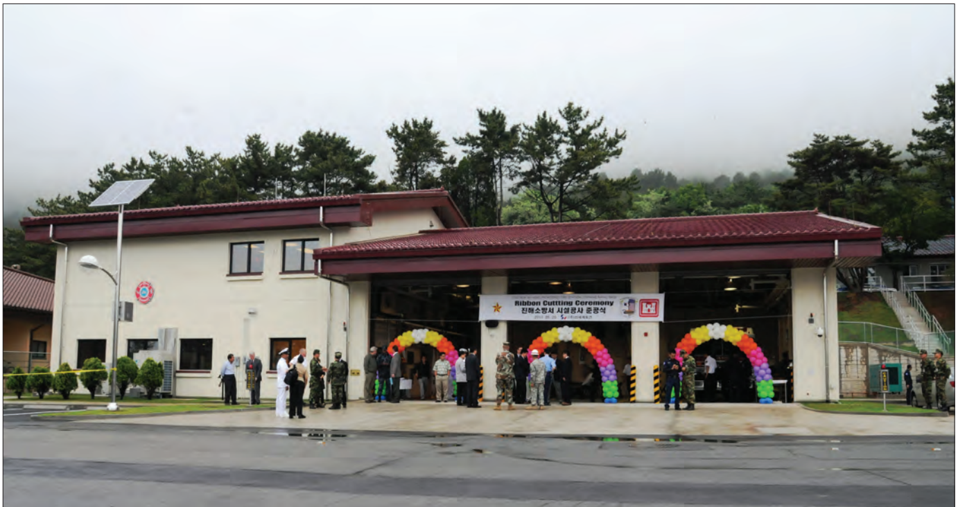
The new fire station at Fleet Activities Chinhae has much more space for both firefighters and trucks than the old fire station, which was over 25 years old. The facility was constructed by Shinsaegye Construction Co., Ltd. using host nation funding. (Photo by Patrick Bray)
