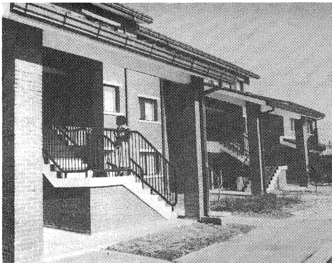
Exterior view of new South Post quarters.
