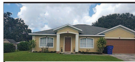
3823 LEEWAY COURT, LAKE PLACID
