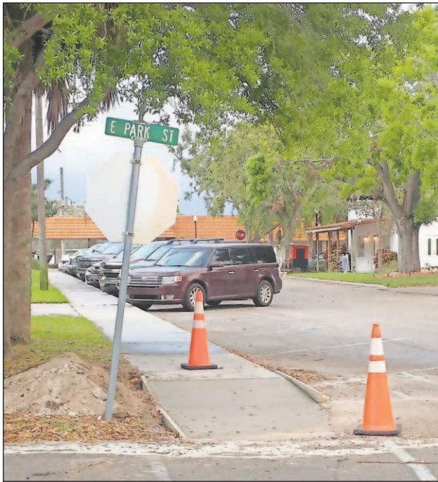
A ramp was installed in an existing sidewalk that previously ended abruptly. This is on the northwest corner of Stuart Park.
