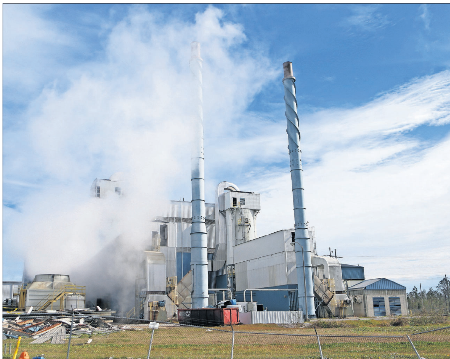
The Bay County Incinerator was temporarily closed after sustaining damage from Hurricane Michael but reopened on Dec. 14. [PATTI BLAKE/THE NEWS HERALD]
