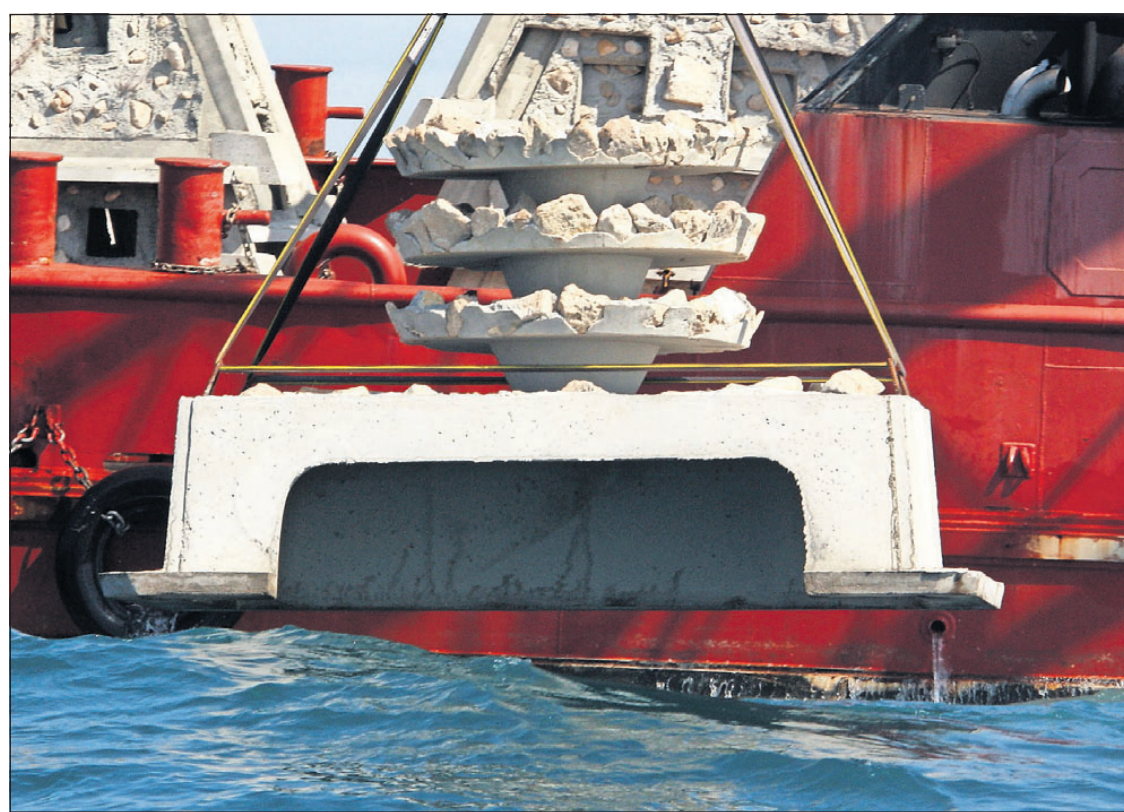
Walter Marine deploys one of nine grouper reef structures sunk last week as part of the Mexico Beach Artificial Reef Association's latest project. [SPECIAL TO THE STAR]
