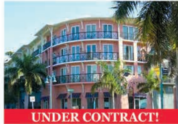
The Astor 235 NE 1st St 509 2 bed/2 bath Penthouse, 2 Parking Spots, Rooftop Balcony w/ Jacuzzi & Ocean view, Italian Marble & Granite in Unit Asking $525,000 Michelle Sadownick 561-633-1020
