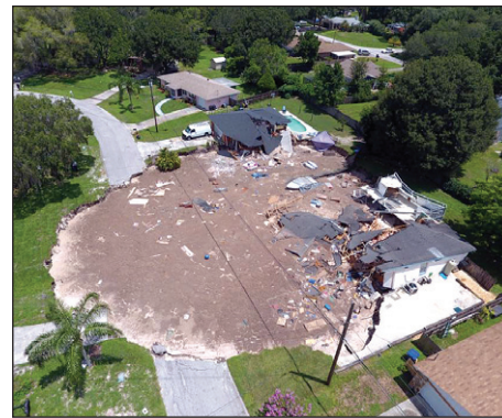
This is an aerial view of a giant sinkhole that developed in Lake Padgett Estates, swallowing two homes and causing several others to be condemned.
