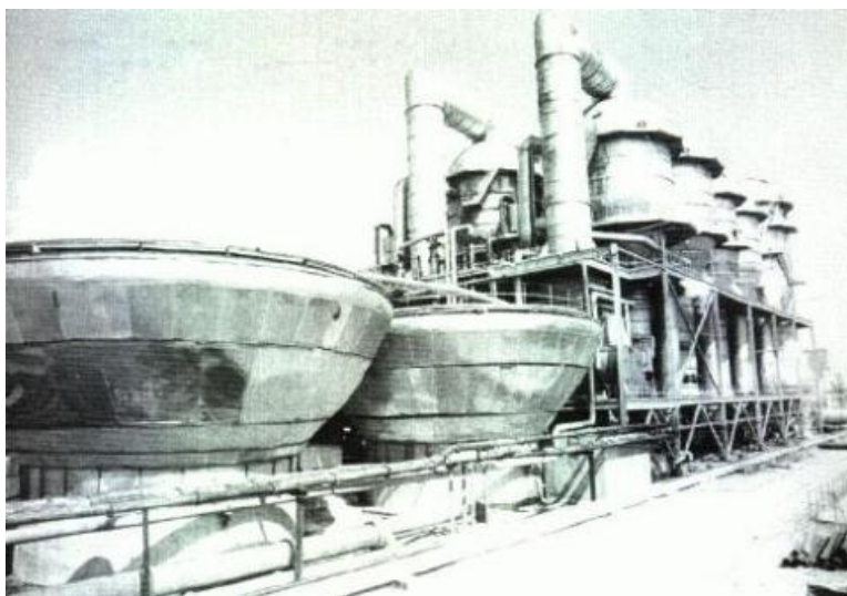
Figure 5.4: Nuclear powered flash distillation desalination equipment located on the Caspian Sea.
