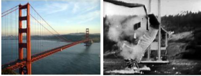
Figure 5.3: The Golden Gate Bridge and the Tacoma Narrows Bridge. The Golden Gate Bridge, a signature landmark of San Francisco, had the world's longest span when opened May 27, 1937. The Tacoma Narrows Bridge, Puget Sound, Washington, broke up after in a strong wind on November 11, 1940.
