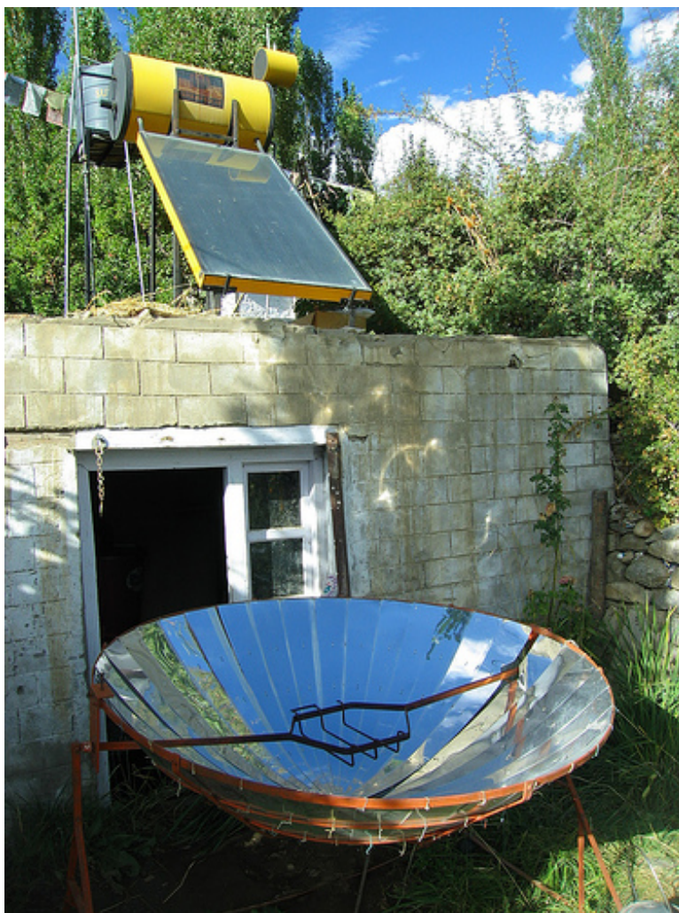
Figure 4.20: A solar cooker and a solar water heater in India. The solar water heater is on the roof of the building. The solar cooker is the silver dish in front of the building.
